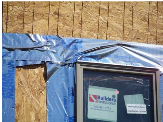
Tape releasing from OSB
