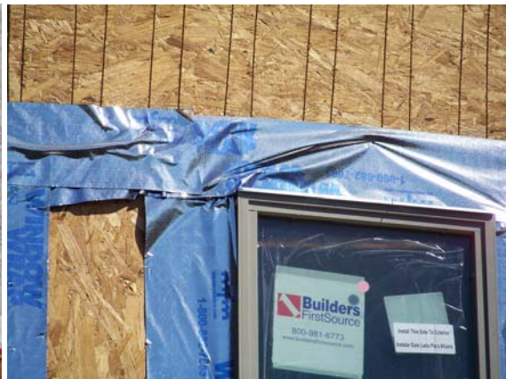
Tape releasing from OSB
